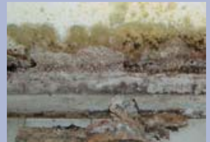
Behind a reference sample cupboard in the warehouse – hidden fungus
